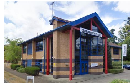
Aspen House Data Centre
