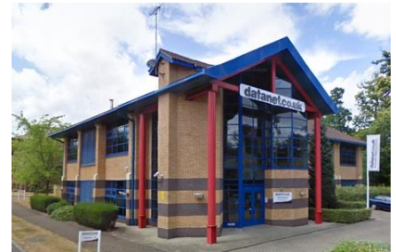
Aspen House Data Centre
